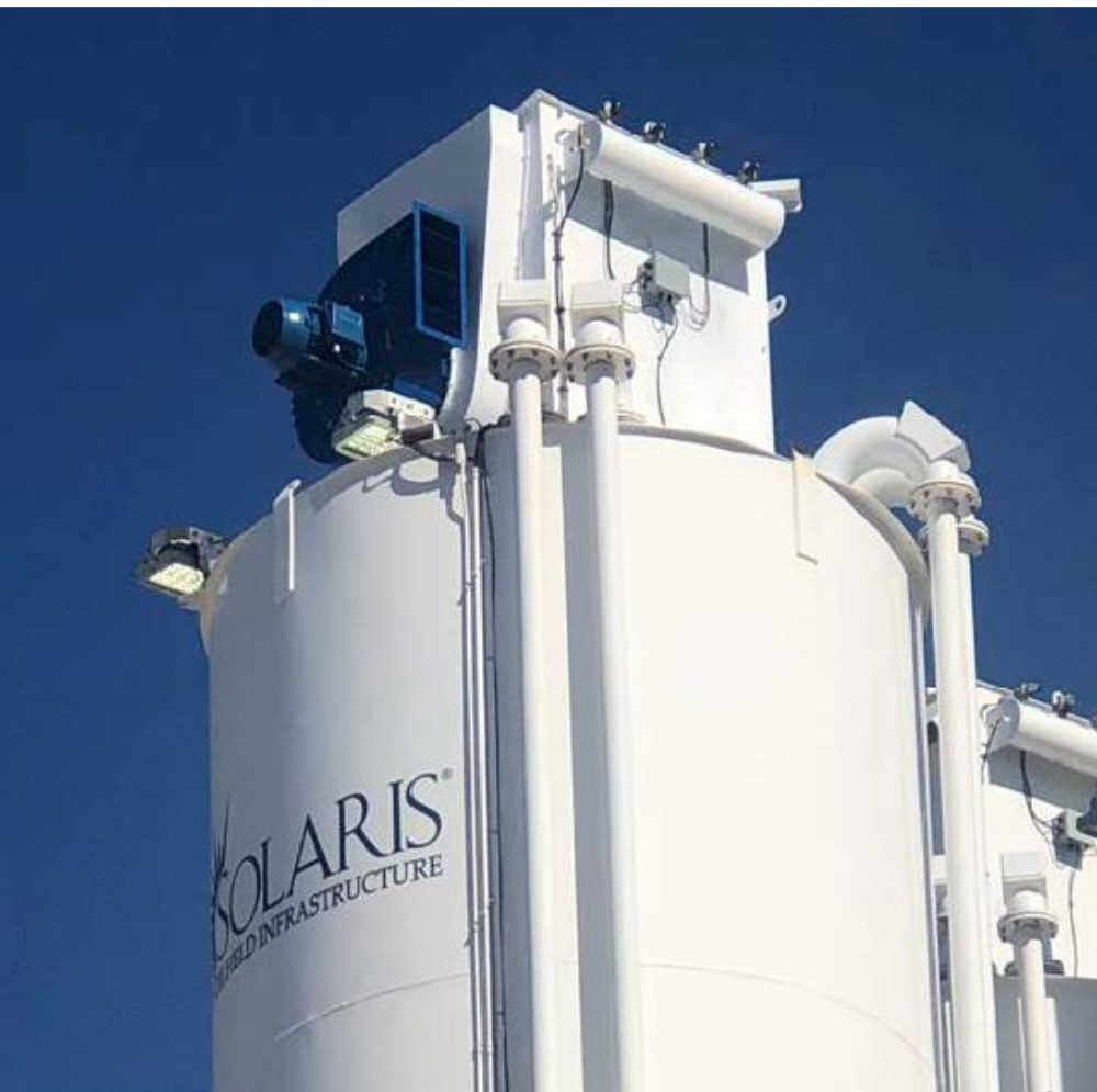
Local Exhaust Ventilation Unit (LEV) with MERV-10 Filters
