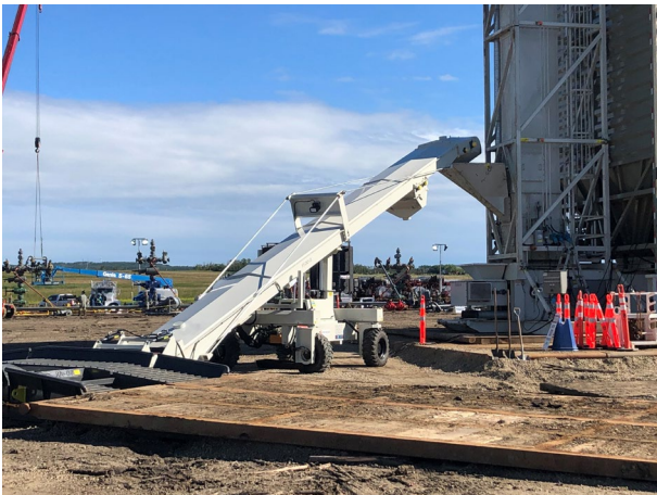
Pics courtesy of Source Energy Services
