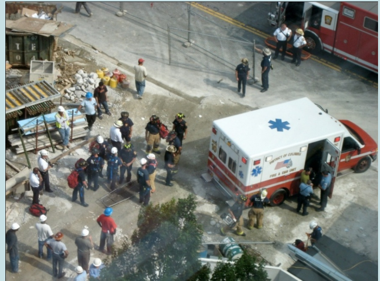
Construction Injury at LEED Gold site Photo: Matt Gillen
