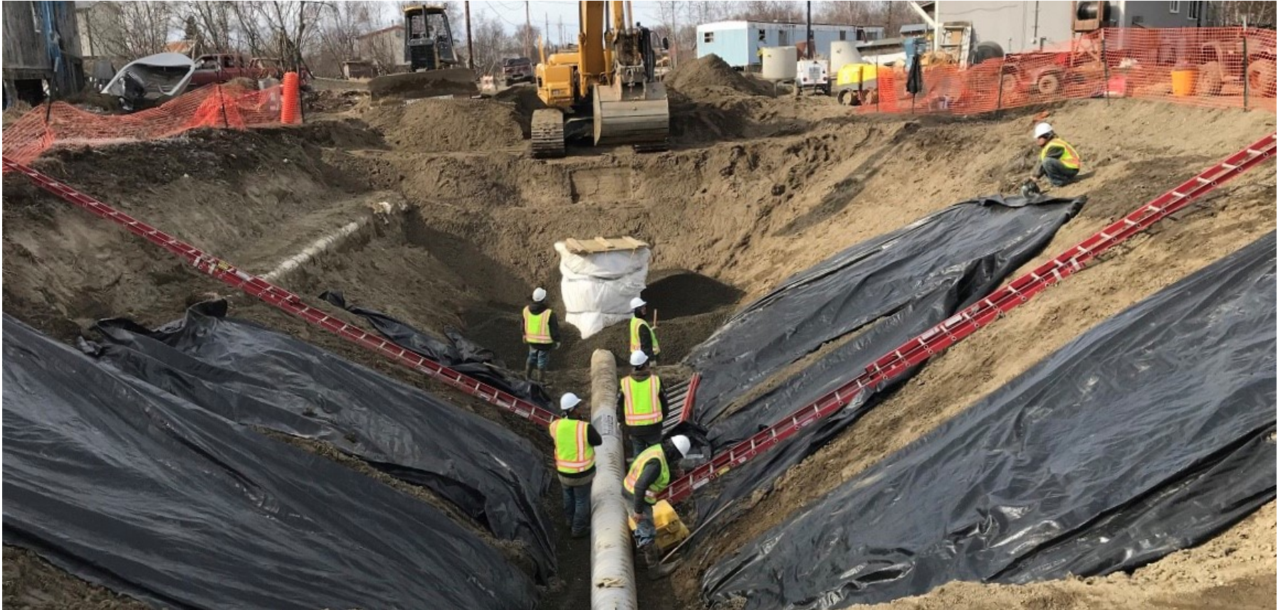
Lower Kalskag, 2018 sewer main construction
